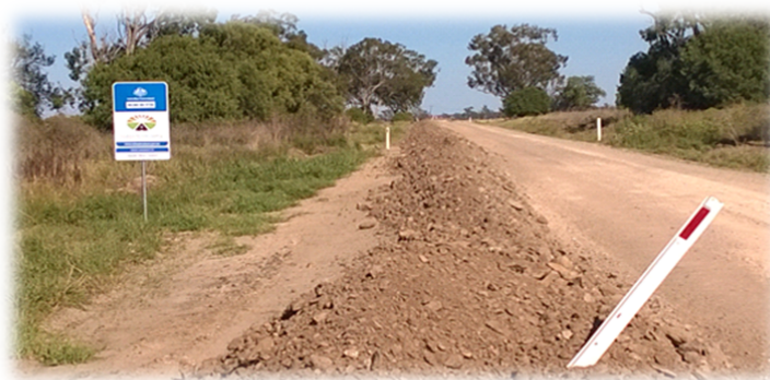
Figure 2 - Gravel Resheeting on SR10 Yallaroi Road
